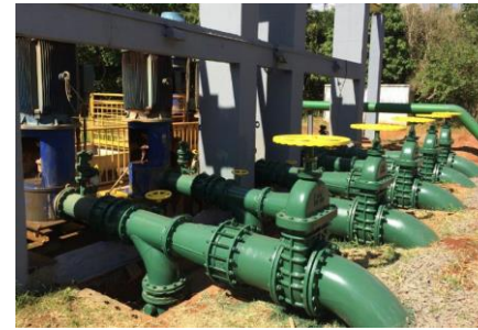
Replacement to energy saving pumps
