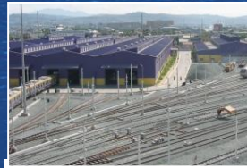
Manila MRT Line 2 Depot
