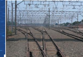
Indonesia Depok Depot
