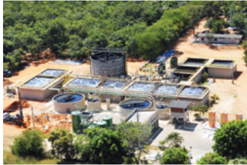
Effluent treatment system. Photo: Cedro Cachoeira/Promotion material.
