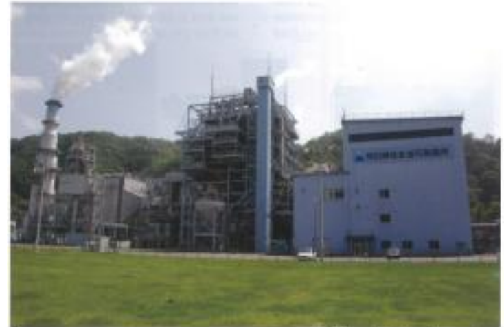
149 MW coal-fired thermal power plant at Kamaishi Works of Nippon Steel & Sumitomo Metal
